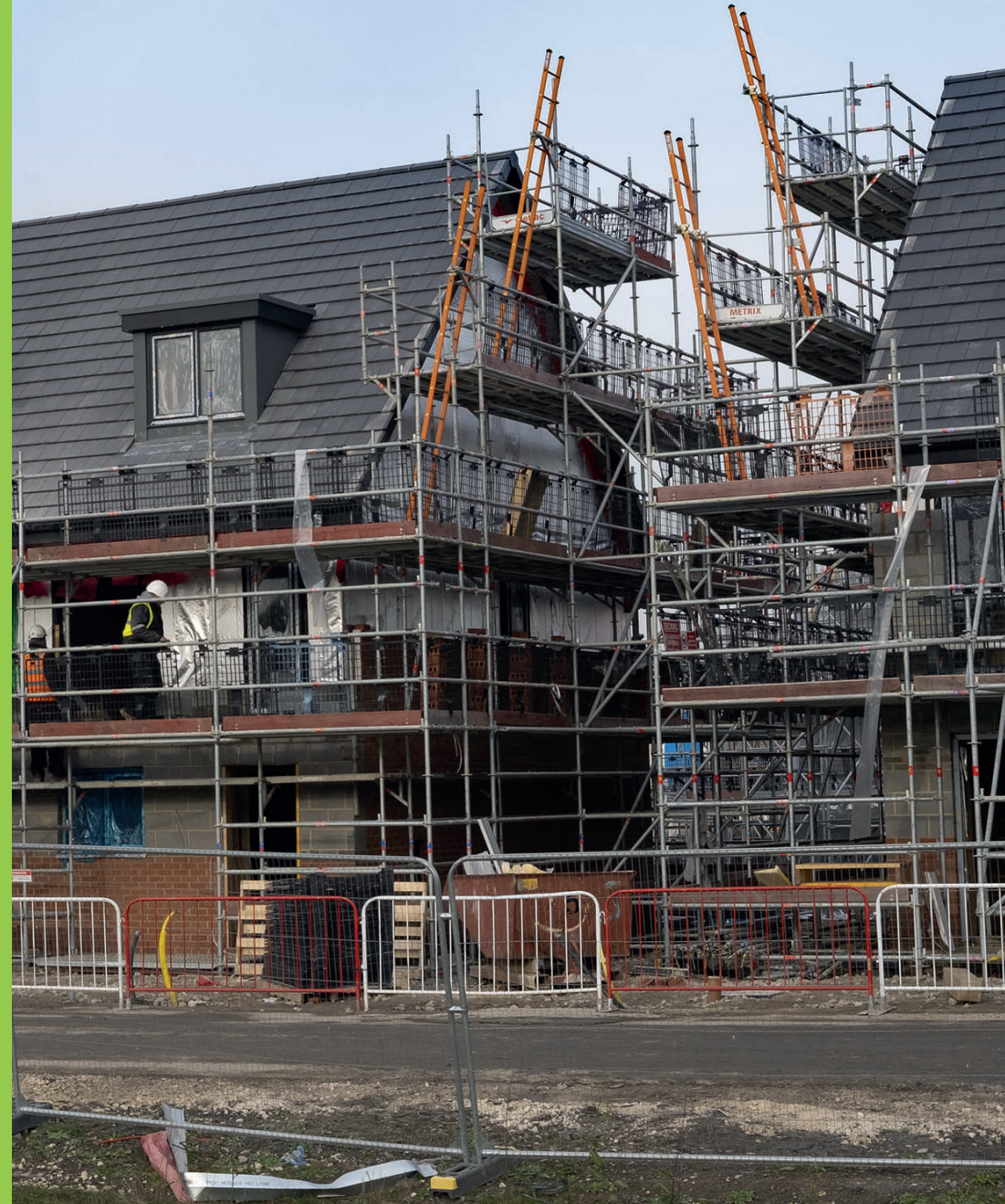
Building energy efficient homes
